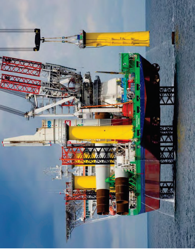
Transition Piece Installation from a Jack-Up Vessel
