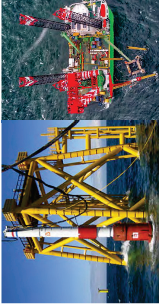
Pile Driving of a Jacket Pile
