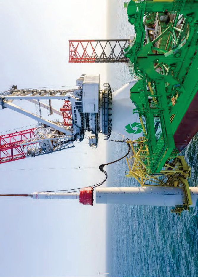
Pile Driving of a Monopile
